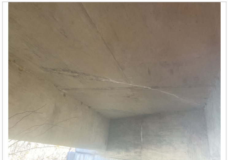
Span # 4. Diagonal cracks with efflorescence in the undersurface.
