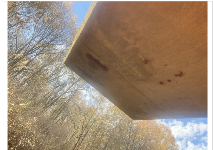
Left overhang of Bent # 2. Spalls with exposed reinforcing.
