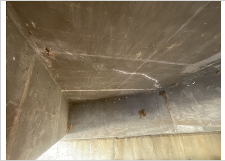
Span # 1. Right. Diagonal crack with efflorescence visible from the undersurface of the top flange.
