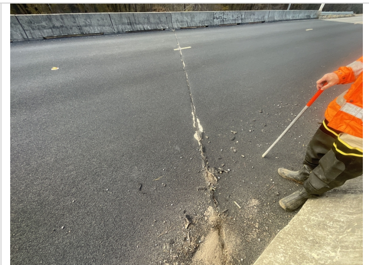
Expansion joint over Bent # 3. Polymer overlay is peeling off of the joint and adjacent deck.
