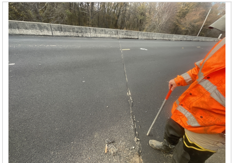
Expansion joint over Bent # 2 polymer overlay is peeling off of the joint and adjacent deck.
