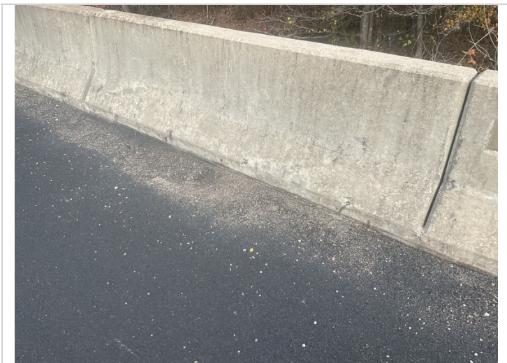
Shallow spalls with exposed reinforcing steel at the base of the parapet.
