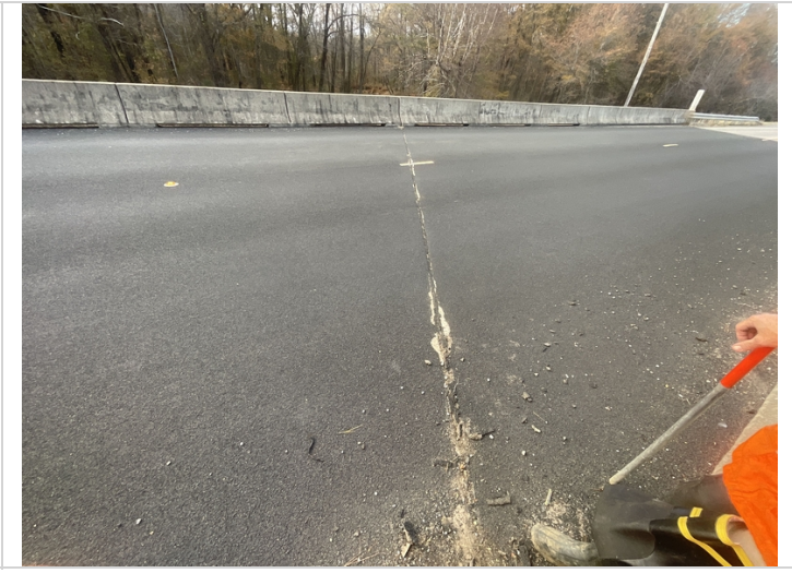
12/01/2022 - JCJ & TJL - The polymer overlay material is peeling off of the joint and adjacent deck.
