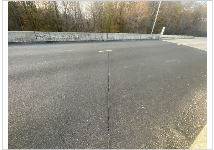
Expansion joint over Bent # 4.
