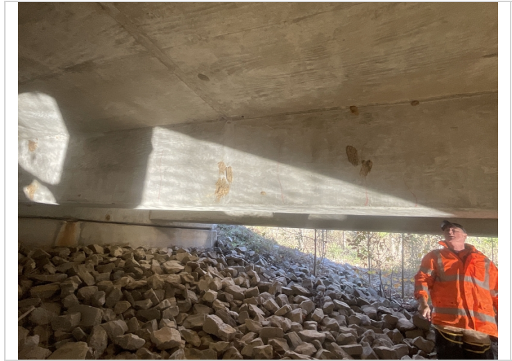
Span 4 - Vertical flexure cracks in the superstructure. Typical.
