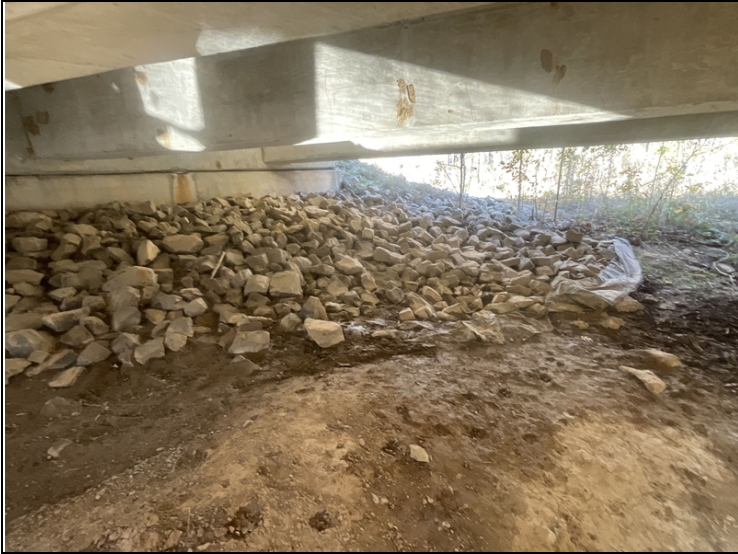
Embankment erosion with exposed filter fabric at the North embankment.
