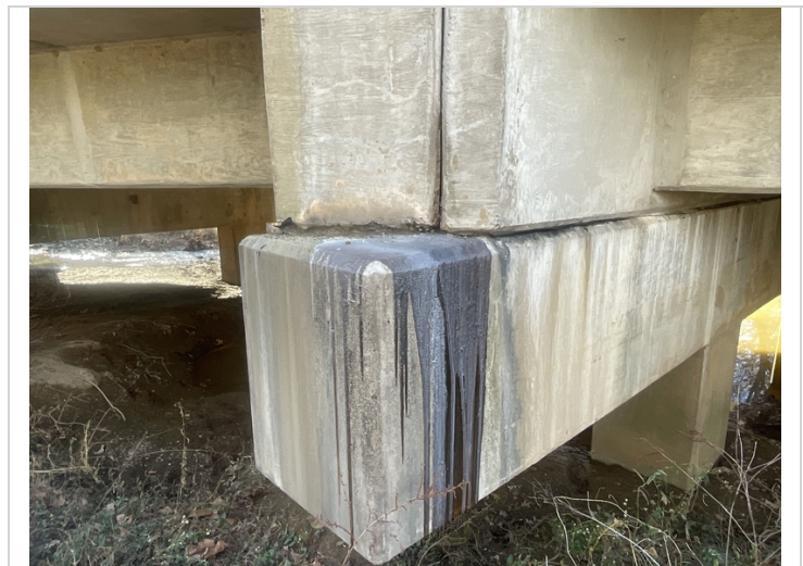
-There is minor concrete deterioration in the exterior edges of the end diaphragms over the intermediate bents. Epoxy leakage on the cap - Right side of Span # 3 over Bent # 4.
