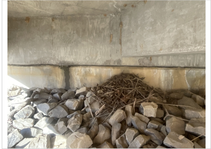
Spalls with no exposed reinforcing steel in the end diaphragm over Bent # 5.
