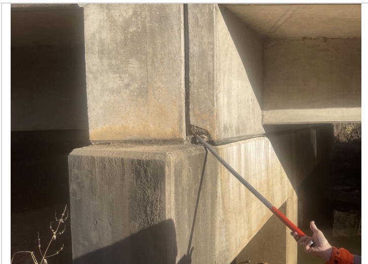
Span # 3. Left end diagram over Bent # 4. Concrete deterioration.
