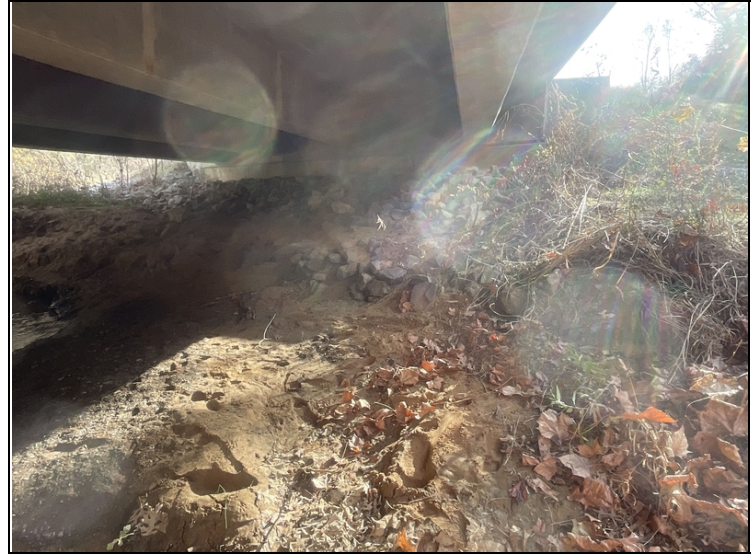
South embankment. Minor erosion.
